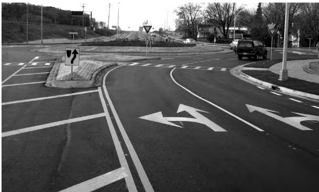
Figure 2-16a: Single white pavement marking separating entry lanes. WIS 30 and Thompson Drive in Madison.
