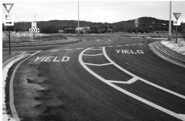
Figure 2-16b: Occasional entry with double white lines separating entry lanes. STH 35 and Hanley Road near Hudson.
